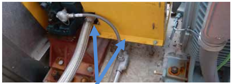
EXAMPLES OF OBSTRUCTIONS THAT WE WOULD NEED TO KNOW ABOUT
